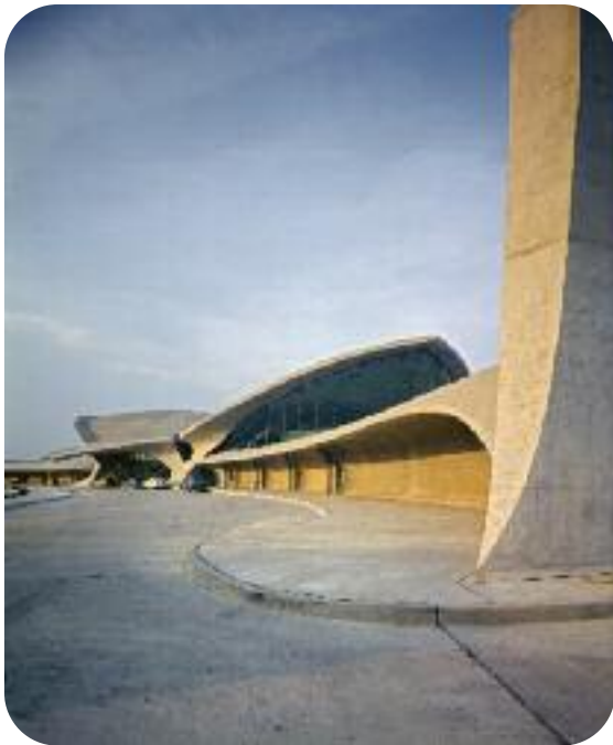
Exterior, TWA Terminal, New York International (now John F. Kennedy International) Airport, New York, circa 1962. Photographer: Ezra Stoller. © Ezra Stoller/Esto.
