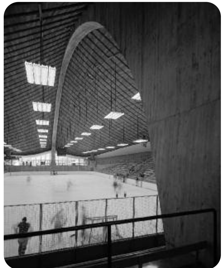
Interior showing structural concrete spine, David S. Ingalls Hockey Rink, Yale University, New Haven, Connecticut, circa 1958. Photographer: Ezra Stoller. © Ezra Stoller/Esto.
